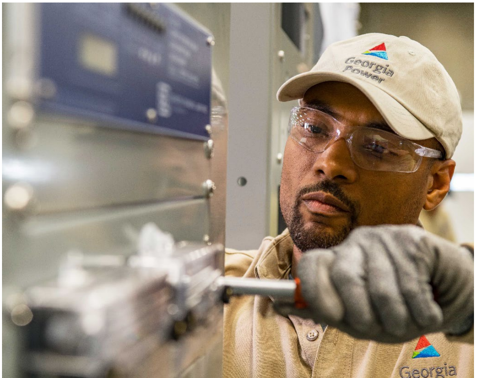
POWER PLANT OPERATIONS
